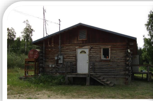
FIGURE 13 TRIBAL OFFICE, FRONT VIEW
