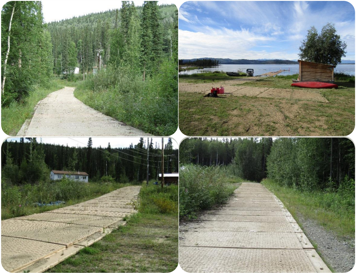
FIGURE 17 DURA MATS THROUGHOUT THE COMMUNITY
